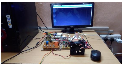
Fig.2. Monitoring the energy meter readings in PC
